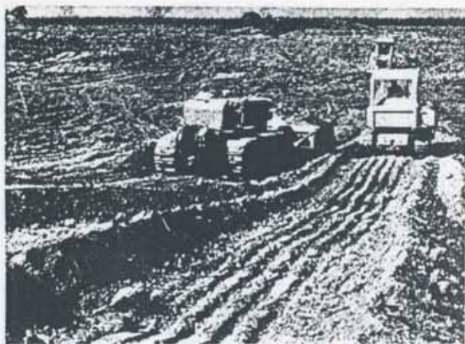
Figure 31. A pond in early stages of construction.
