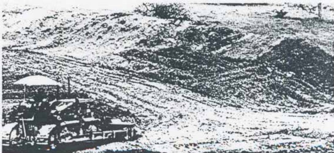
Figure 32. Sod and topsoil are stockpiled for later use.
